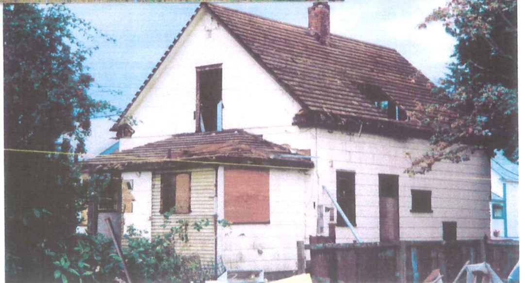
REAR VIEW (NE CORNER)
