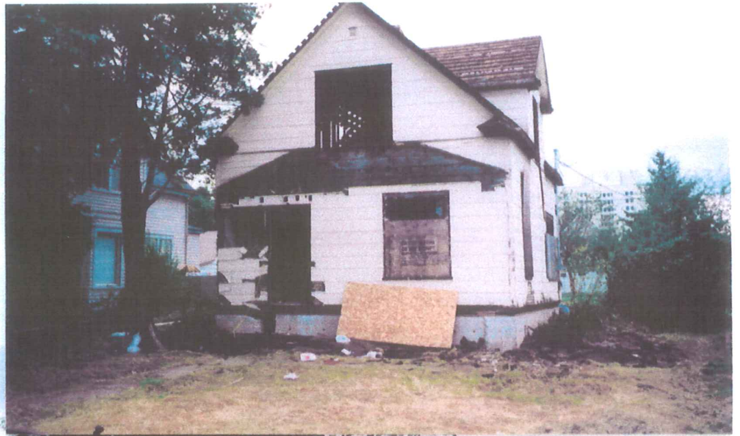
FRONT VIEW (WEST SIDE)
