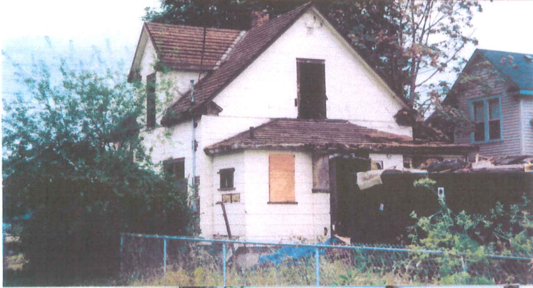
REAR VIEW (SE CORNER)
